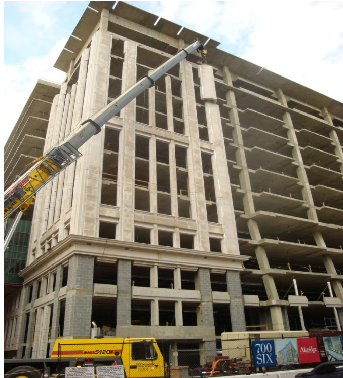
Picture 2.1-Concrete Superstructure
